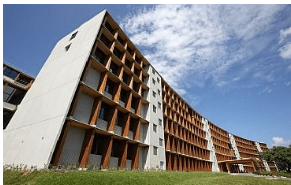
Photo credit: Steeltech Industries PTE Ltd
