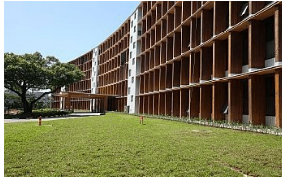
Photo credit: Steeltech Industries PTE Ltd
