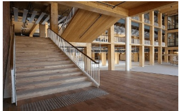
Photo credit: Steeltech Industries PTE Ltd
