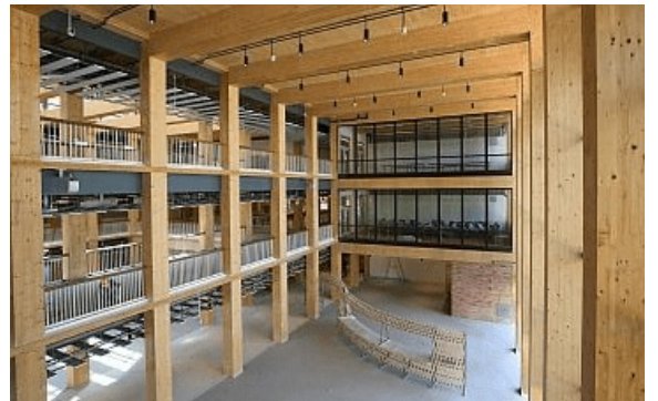
Photo credit: Steeltech Industries PTE Ltd
