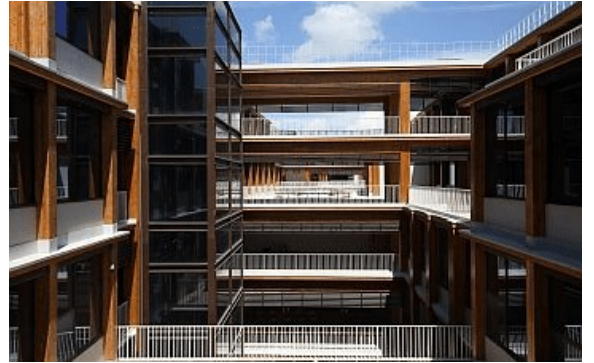
Photo credit: Steeltech Industries PTE Ltd
