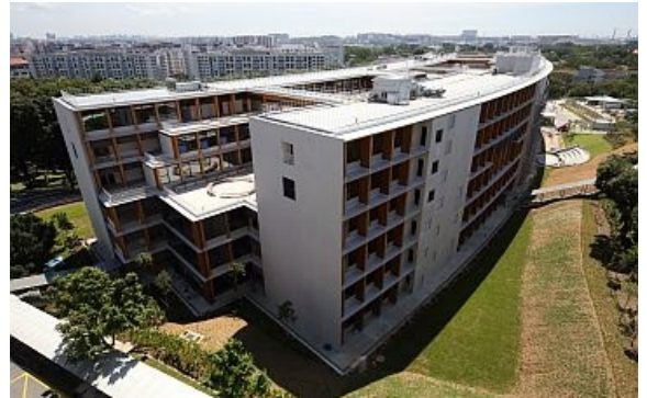
Photo credit: Steeltech Industries PTE Ltd
