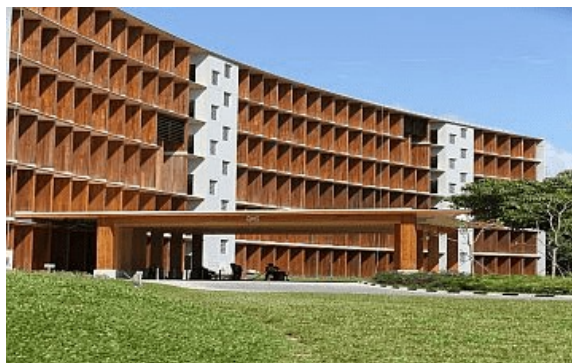
Photo credit: Steeltech Industries PTE Ltd
