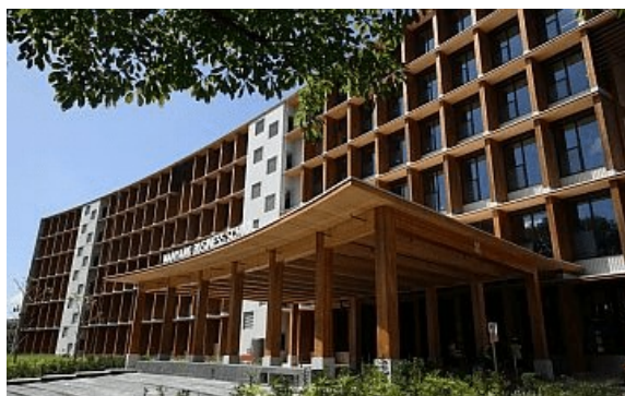
Photo credit: Steeltech Industries PTE Ltd
