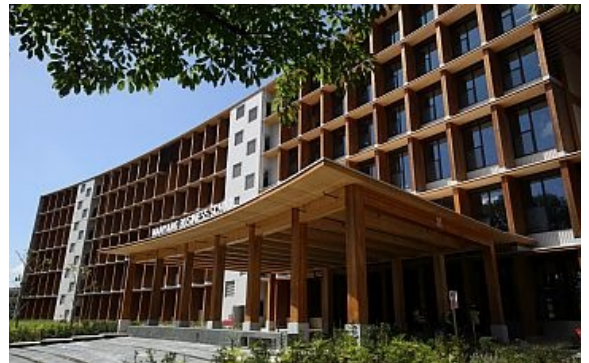
Photo credit: Steeltech Industries PTE Ltd
