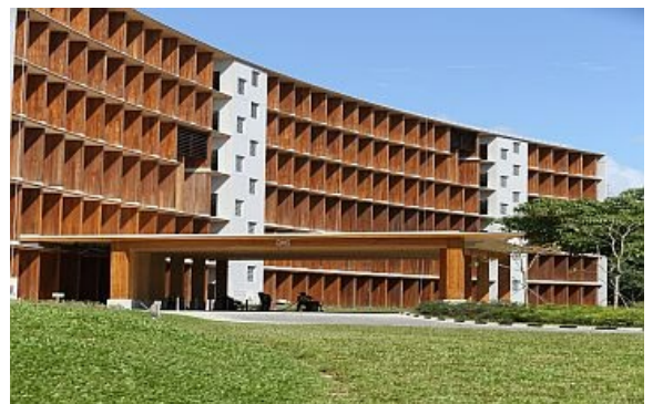
Photo credit: Steeltech Industries PTE Ltd
