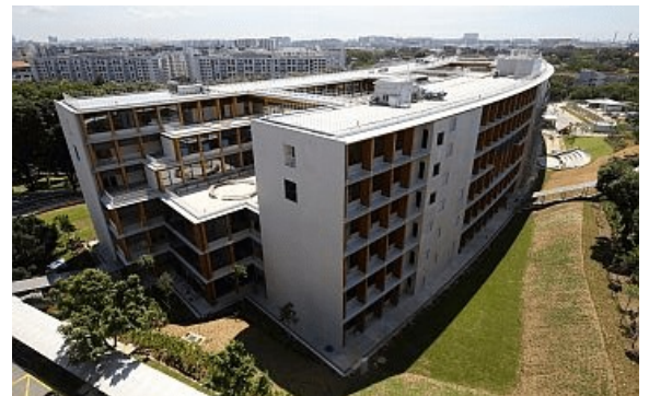
Photo credit: Steeltech Industries PTE Ltd
