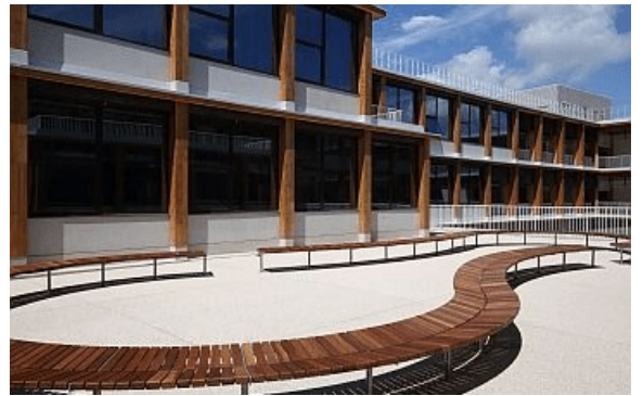
Photo credit: Steeltech Industries PTE Ltd
