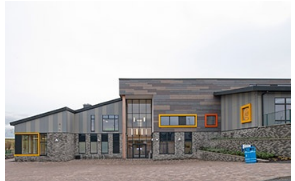
Photo credit: Aberdeenshire Council
