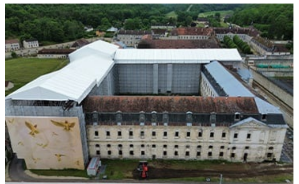
Photo credit: ©Cruard Charpentres
