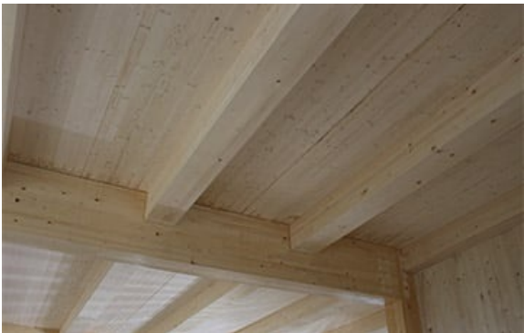
Photo credit: B&K Structures
