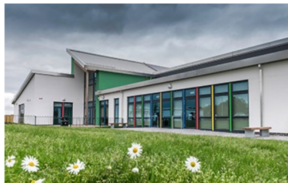
Photo credit: G-Frame Structures / Aberdeenshire Council
