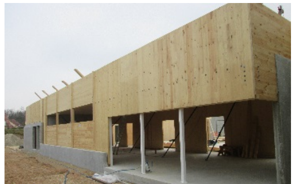
Photo credit: Aux Charpentiers de France
