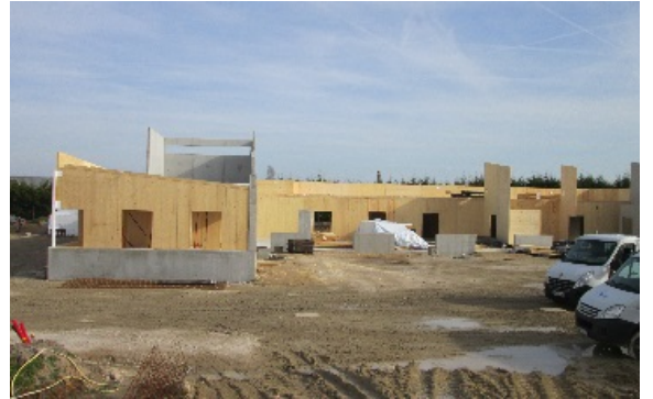
Photo credit: Aux Charpentiers de France
