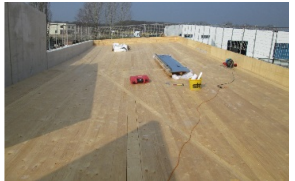
Photo credit: Aux Charpentiers de France
