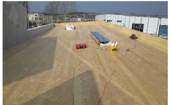
Photo credit: Aux Charpentiers de France
