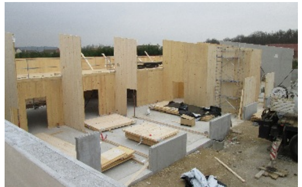
Photo credit: Aux Charpentiers de France
