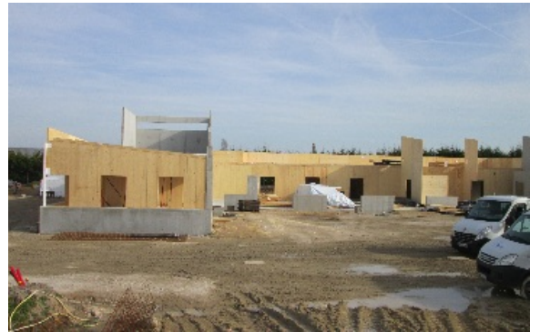
Photo credit: Aux Charpentiers de France
