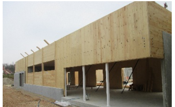
Photo credit: Aux Charpentiers de France
