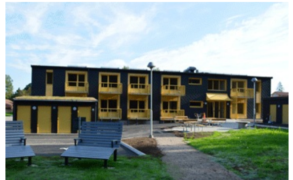
Photo credit: Nock Massiva trähus
