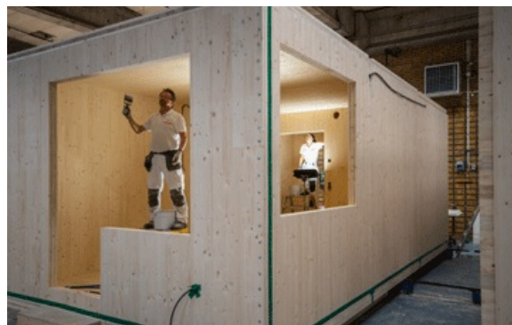
Photo credit: Nock Massiva trähus
