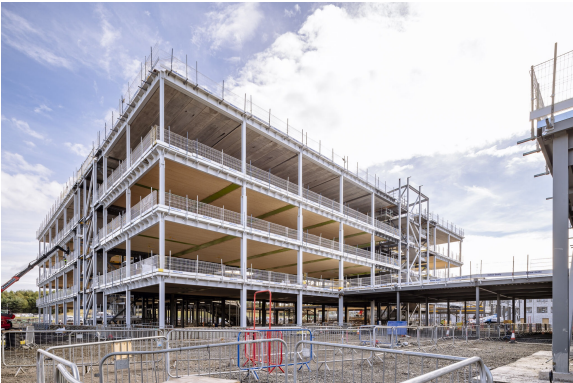
Photo credit: B&K Structures
