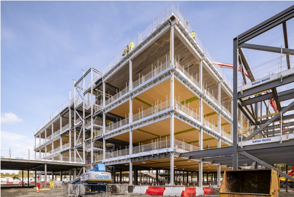
Photo credit: B&K Structures
