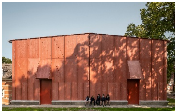
Photo credit: Jim Stephenson Photography
