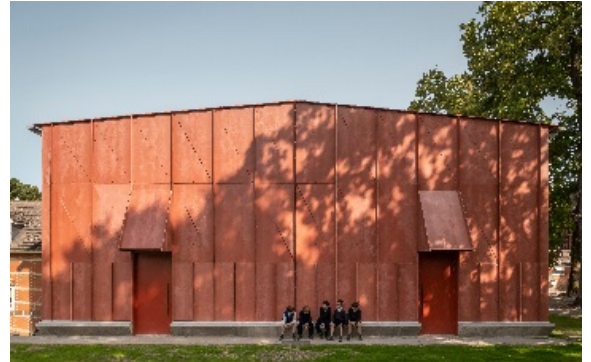
Photo credit: Jim Stephenson Photography
