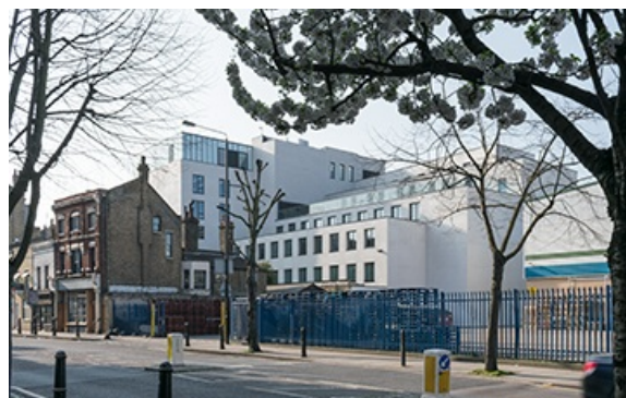
Photo credit: Jim Stephenson Photography
