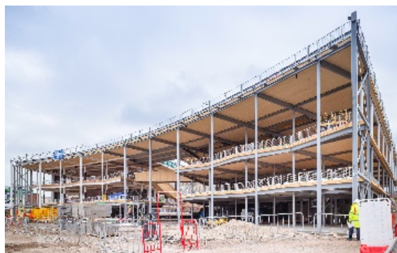
Photo credit: B&K Structures
