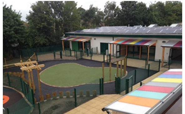
Photo credit: The Bridge School
