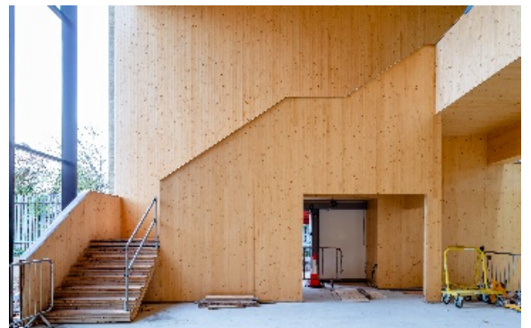
Photo credit: B&K Structures
