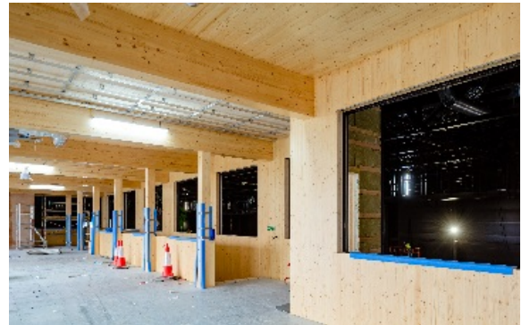
Photo credit: B&K Structures
